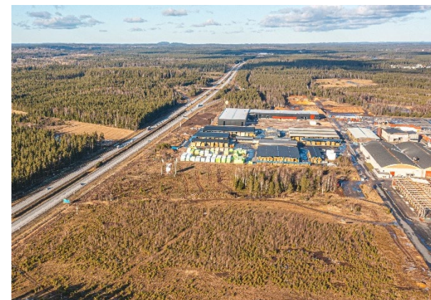
Vaggeryd Logistics Park adjacent European Highway E4, south of Jönköping
